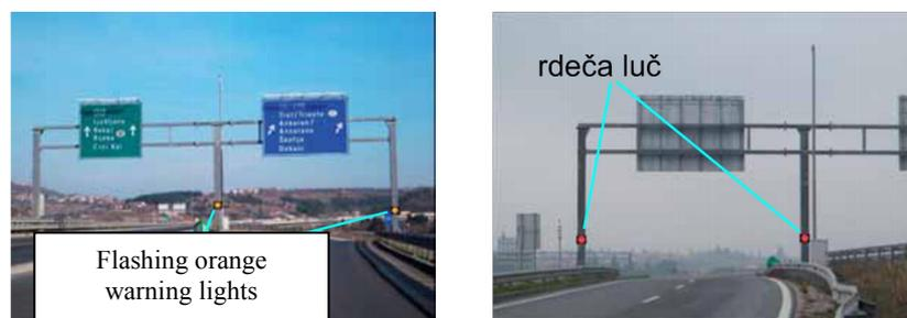
**Figure 5:** Warning signalization on exit ramp (left for correct-, right for wrong-way driving motorists)
